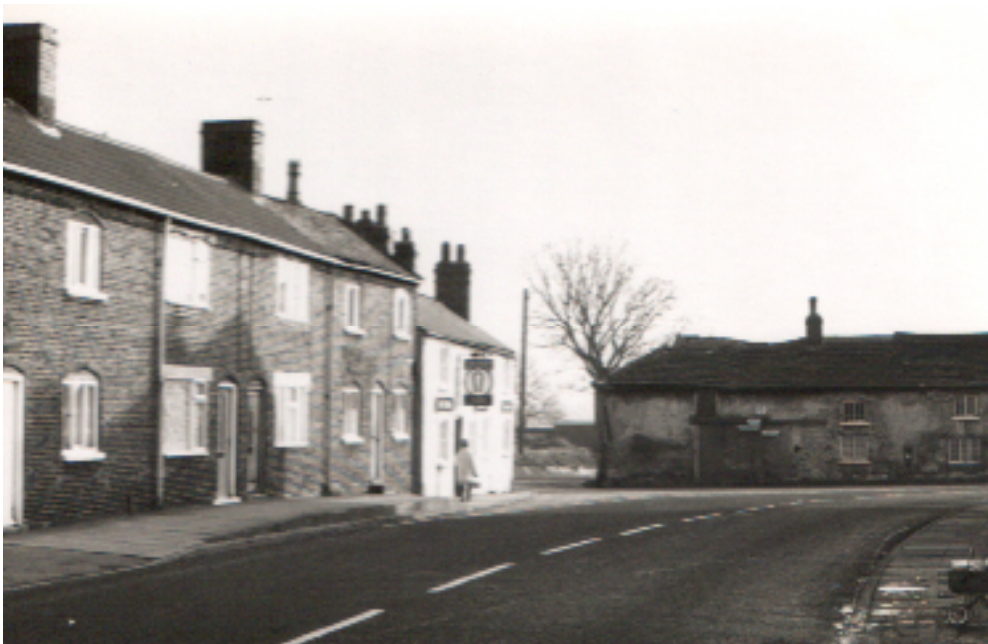
Main Street, Barwick with the New Inn and Glebe Farm (demolished 1973)
