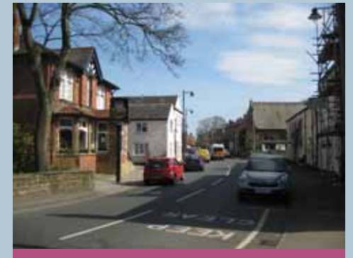
Main Street is a main through road and as such has high levels of vehicular activity.
